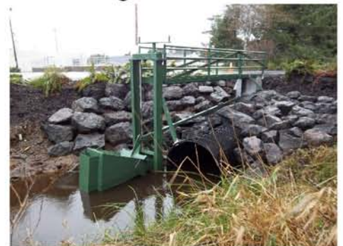
NSG5ra Tidegate Installed
