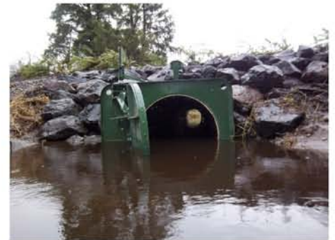
NSG5ra Tidegate Installed
